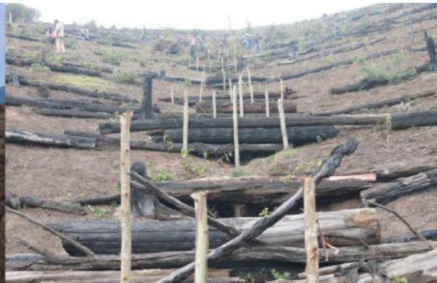
Fig. 2. Gully plugging using wattle logs
