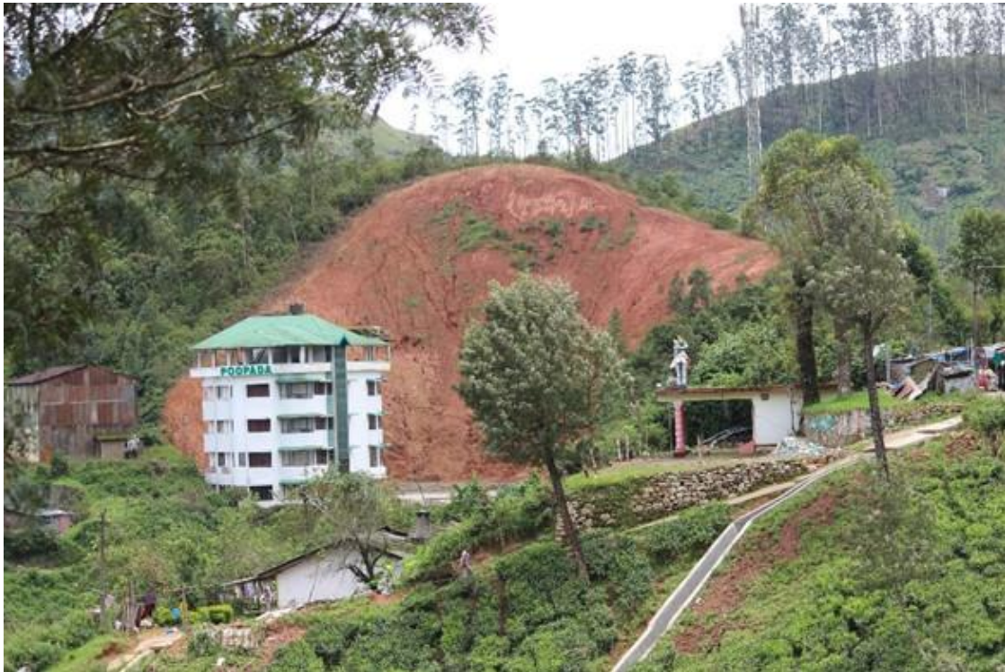
Fig. Landslide at Munnar Grama Panchayat
