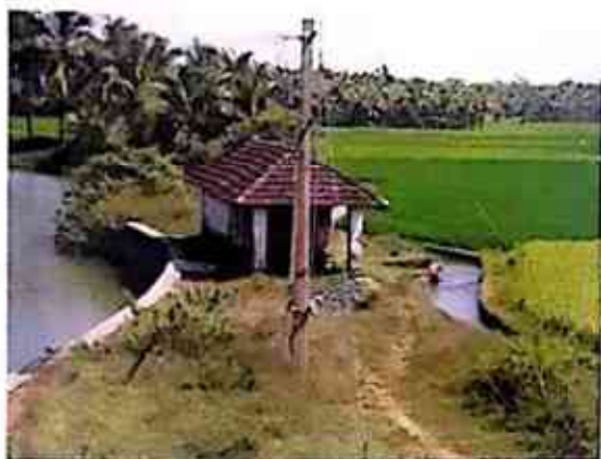
Fig. 48 A pump huse at Pathramangalam
