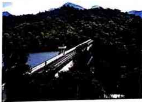
Fig. 12 Peppara Dam © The Hindu
