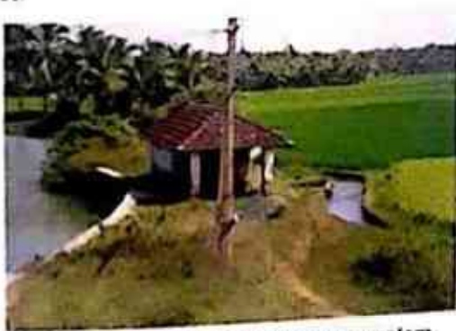
Fig. 13 A pump house at Pathramangalam
