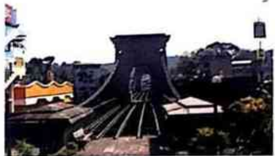
Fig. 02-11 Wooden bridge at Punalur
